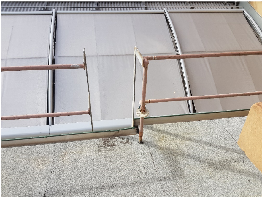
Figure 6: Balustrade North West
