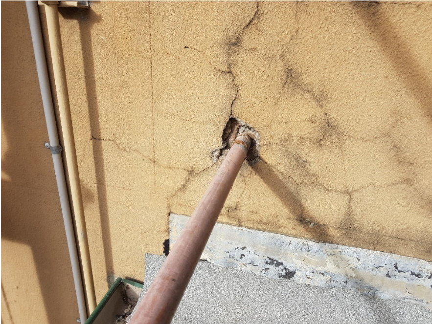
Figure 7: North West Balustrade Closest to Central Dome Fixing
