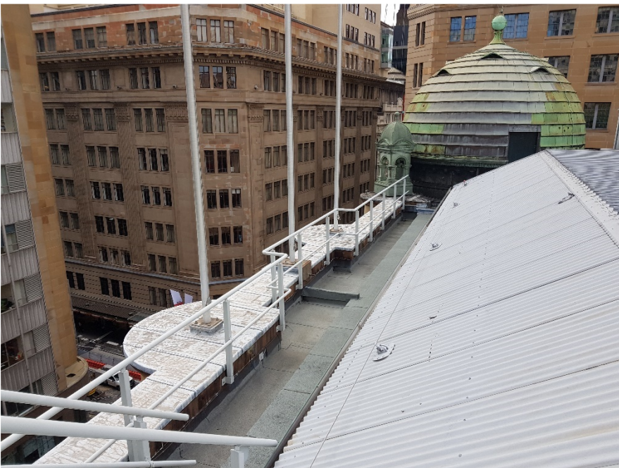
Figure 2: Flag Poles North End
